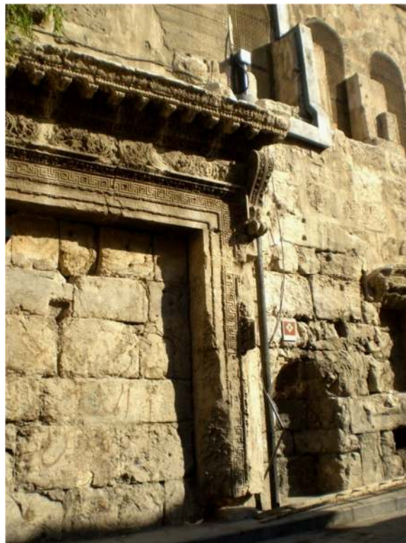
The southern door of the inner temenos of the Jupiter Temple as part of the Great Umayyad Mosque's qiblah wall facing the south. When the Church of St John the Baptist was shared by Muslims and Christians, this door functioned as the main entrance to the building. Upon entering the Church, the Christians turned to the left (the west) to go to their section of the Church, and the
